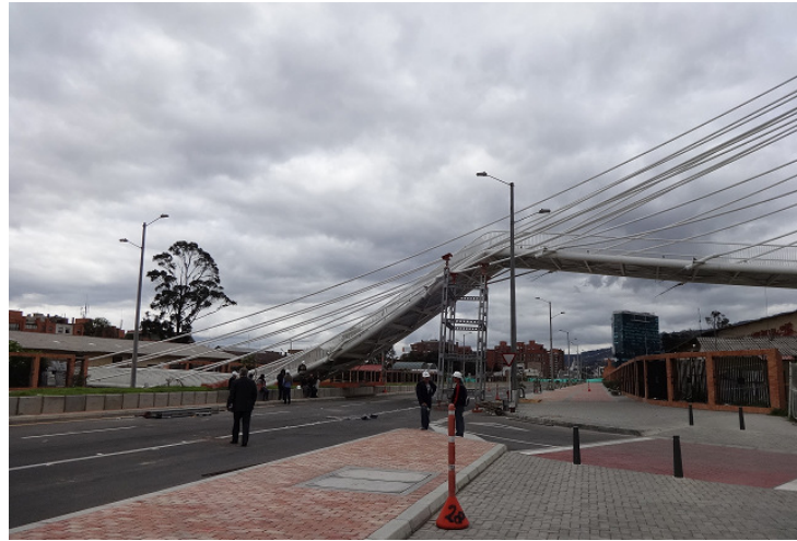
Photo 1. Failure of Cantón Norte Bridge. Source: Photo by Zulma S. Pardo V.
